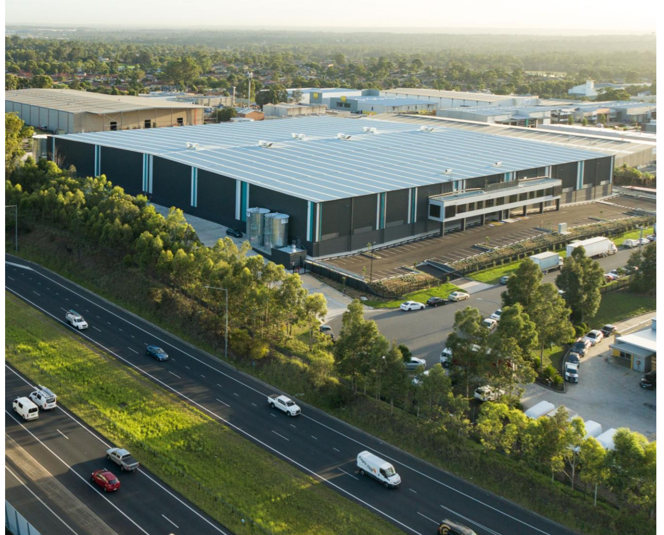
42 Cox Place, Glendenning, NSW.
