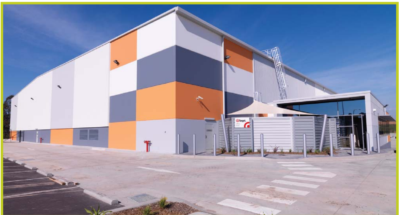
connect@erskine Park - Target Facility
