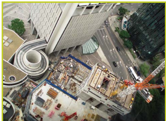
Construction shot: One One One Eagle Street, Brisbane
