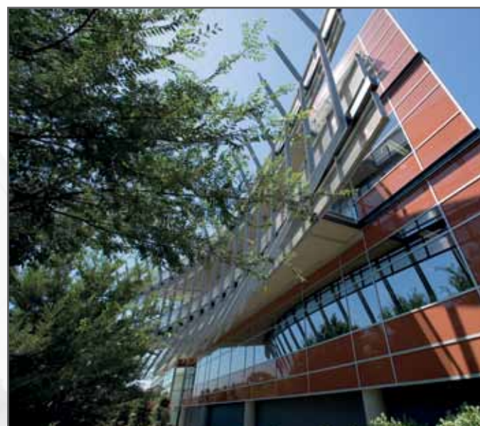
QUAD BUSINESS PARK, SYDNEY OLYMPIC PARK, NSW
